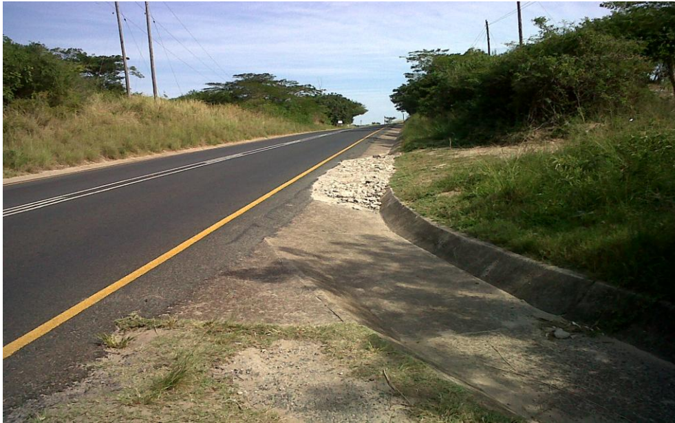
Building rubble being placed on a R22 storm water drain to make unauthorised access.
